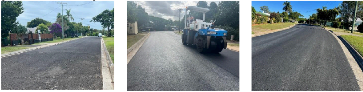
Figure 1 - Site 1 before, during and after construction.
