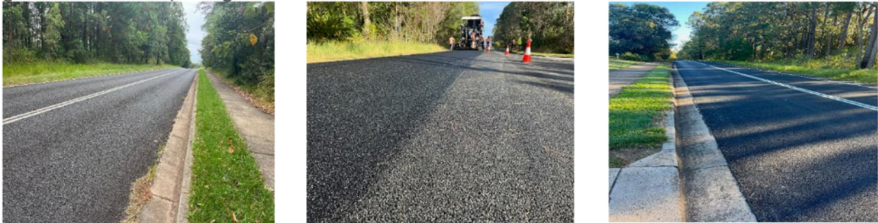
Figure 2 - Site 2 before, during and after construction
